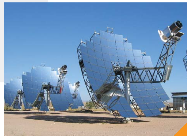
CSP Dish Systems
