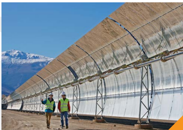
Parabolic Trough System
